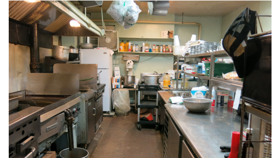
Existing kitchen facilities have been in use for 70 years with piecemeal updates.
