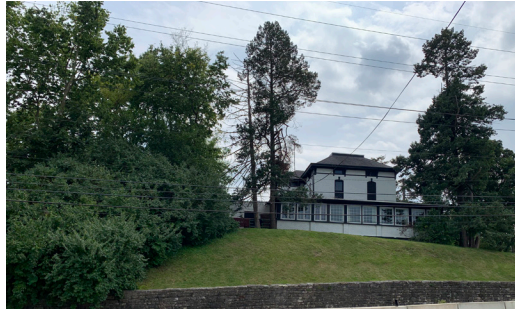
South side elevation showing existing unsympathetic vestibule and restroom addition.
