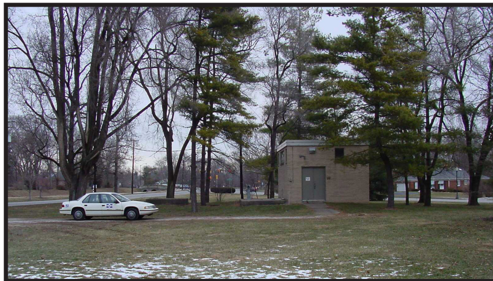
View to North of Lift Station and Access Drive
