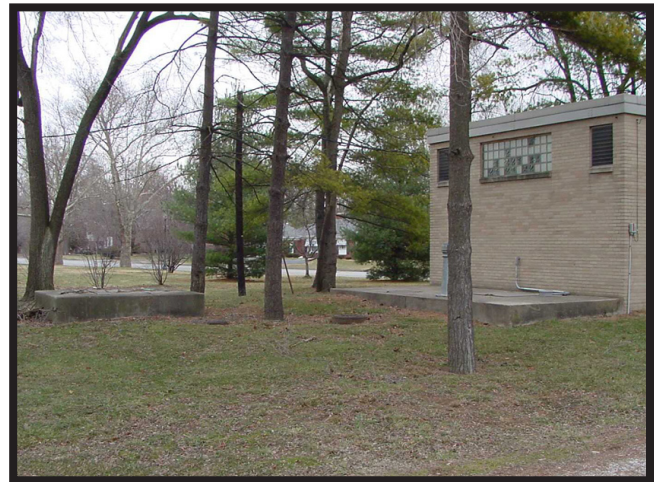
Lift Station and Associated Manholes
