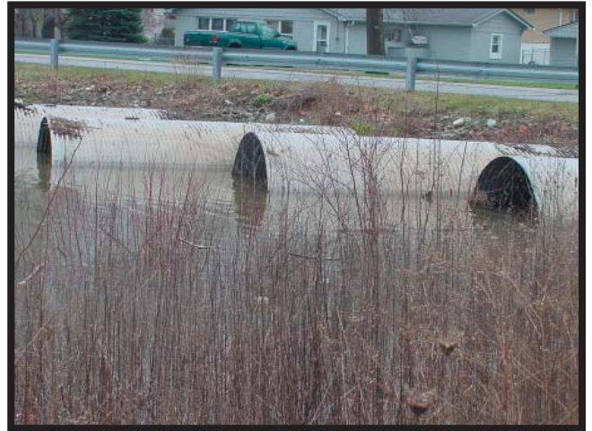
East Parcel facing East
