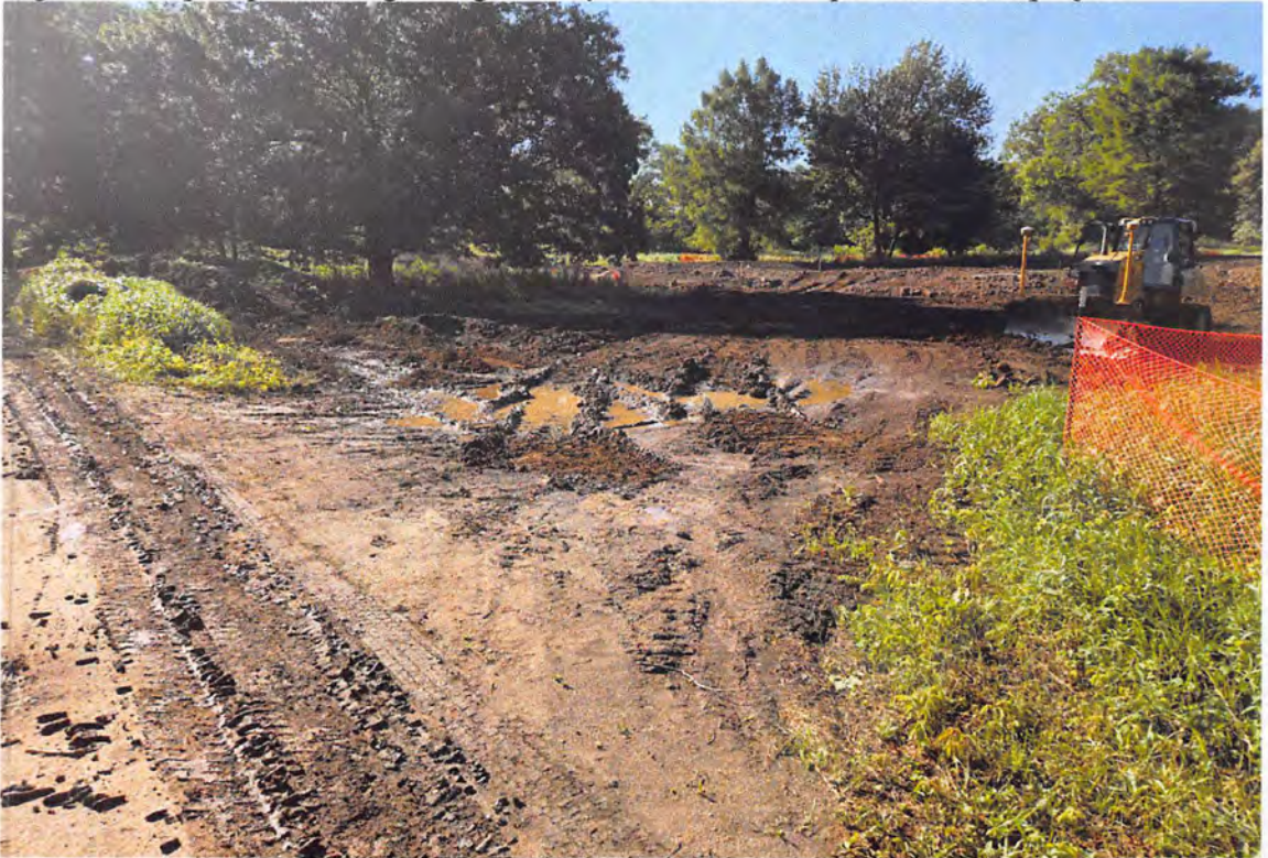
Figure 11. Active construction in the southern portion of the project.
