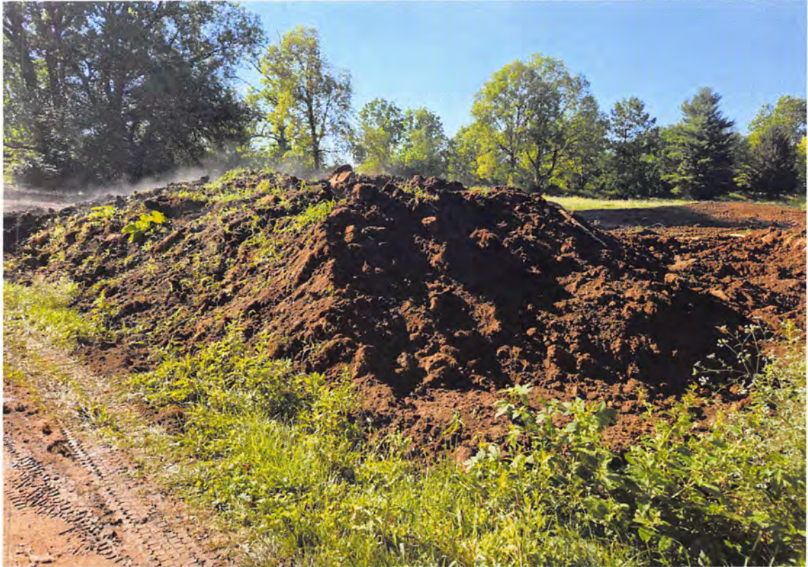
Figure 12. Another spoil pile in the southern portion of the project.
