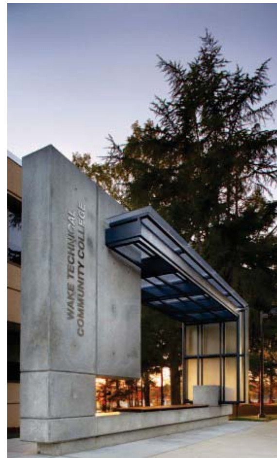
Bus Shelter, | Wake Technical Community College | Raleigh, NC
